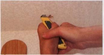
First of all, check that there are no obstructions inside the caravan where the switches are to be fitted. Dealing with the illuminated switch first, drill a pilot hole through from the outside; one of the spare fixing holes in the light's backplate is ideal. Open the hole up to 6mm. Inside the caravan, use the template which comes with the switch as the guide for cutting the wallboard and insulation.
