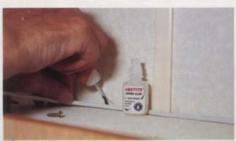
Rather than use two separate cables, I opted for a length of 3 amp mains lighting cable because it had a white outer sheath, which I felt would be less obtrusive. Having connected the brown lead to the live terminal on the light and the blue to the return, I fed the cable through the hole into the caravan and routed it to the reading light on the underside of the forward roof locker. I used Superglue to secure the cable in position.
