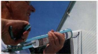
It's almost certain that you won't be able to use the original screw holes to secure the PIR light. Although the gasket will probably cover them, I believe in a belt and braces approach and so squirted mastic into the holes
