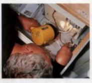
3 I needed a hand lamp to check which MCB (micro-circuit breaker) had the existing charger connected to it (above). As we suspected, it was the 6A MCB. I already knew from my original checks that both MCBs were working satisfactorily and current was getting to the original charger.
