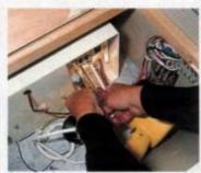
5 The next job was to fit shrouded spade terminals to the live and return leads from the charger to the battery terminals. Whenever possible, use a purposedesigned stripping tool which removes the insulation without damaging or cutting the
