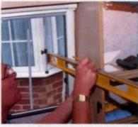
Probe the pilot hole with a piece of coathanger wire and then transfer the position of the hole on to the cupboard wall.
