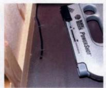
The cable is stapled down the wall and to the floor to the 6mm exit hole.
