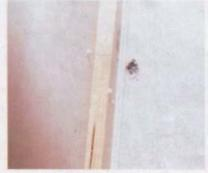
Carefully drill through the cupboard wall; and, when you have confirmed that it lines up with the hole through the framework, open it up to 10mm dia.
