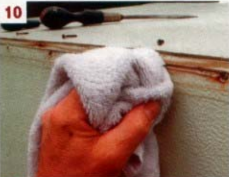
10 ■ Turps substitute seemed to help in the cleaning-up process, but it took quite a time to completely tidy up the surface
