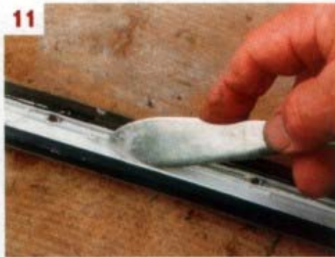
11 ■ An old fish knife is my favourite tool for getting into tight spaces such as removing sealant from the rear side of the channelling
