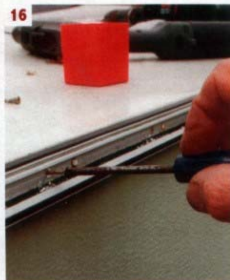
16 ■ Once the new holes had been finally prepared with a countersink, the new screws were driven home
