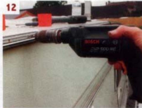
12 ■ The channel was temporarily re-fixed so that fresh holes could be drilled to receive replacement screws
