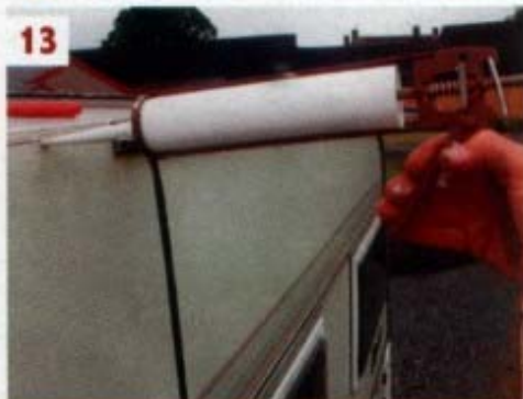
13 ■ Sealant was pumped into all the holes, both the original ones and the new holes for replacement fixings
