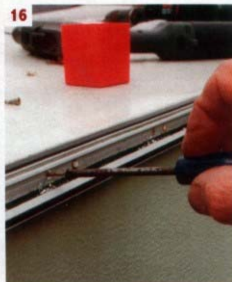
16 ■ Once the new holes had been finally prepared with a countersink, the new screws were driven home
