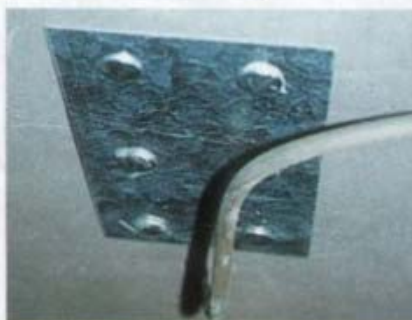
4 The underfloor plate and coachbolts make it highly unlikely that anyone could remove the safe without first cutting the floor away.
