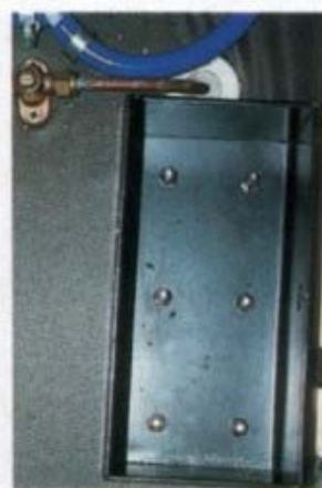
3 The safe body was secured using the Nyloc nuts.
