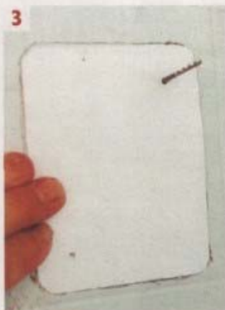
3. Drill two holes in the sidewall leaving one drill bit in place
