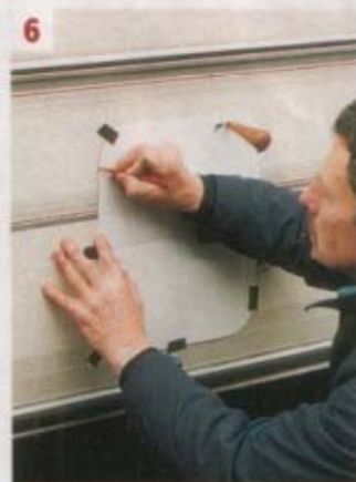
6. Positioning the template correctly is extremely important
