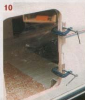
10. A wooden frame fits inside the void and is bonded in place
