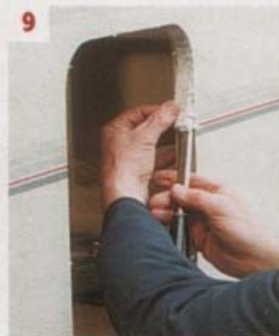
9. Strengthen the aperture by cutting away the wall's insulation
