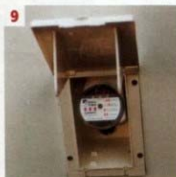
9 Having reconnected the mains, I tested the circuit with a test plug. Neons lights meant all was OK
