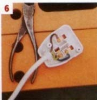
6 After removing the excess mastic I connected a length of 13 amp three core cable to the socket
