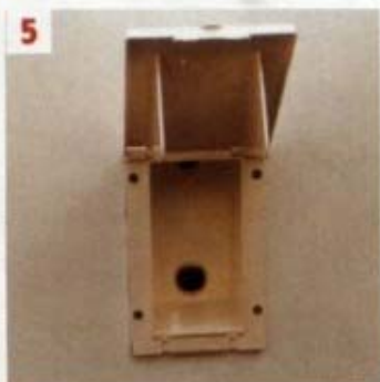
5 No. 6 x 5/8in long stainless steel screws were used to secure the socket housing in position
