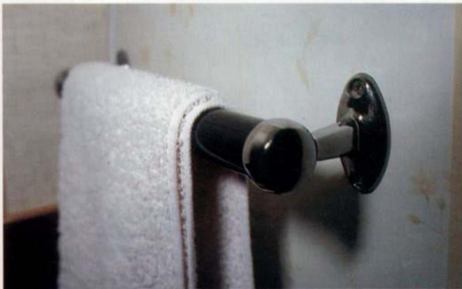
Substantial towel rails like this (above) need equally substantial screws to affix them successfully to inner caravan walls.
