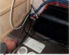
8 You will need to run a 12V supply for the electronic ignition of the new fridge. I used scotchloks to connect to the 12V auxiliary circuit. When connecting the cable, make a note of which is the live lead as ignition polarity is important.
