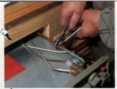
G Use two spanners to undo the compression fitting at the gas pipe joint. By using two spanners you are much less likely to damage either the fitting or, more importantly, the copper pipe. The same applies when tightening any compression fitting.
