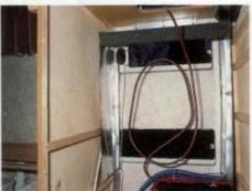
Use a couple of small screws to fix the installation box to the wall. Then bend the sides inwards slightly so that they will fit firmly against the sides of the fridge. Once the box is secure, make sure there are no kinks which could prevent the fridge from fitting snugly.
