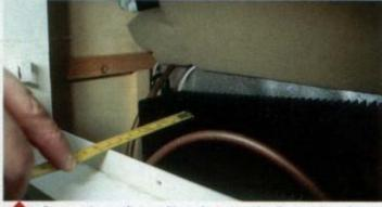
Remove the ventilator grills and measure the distance from the wall to the cooling unit on the RM 4230. If it is any less than 85mm, you will not be able to fit the RM 4271. See 'next step' for the reason why.
