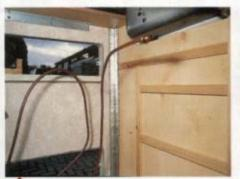
After I'd removed the fridge, I could see that there were gaps between the wall and the sides of the fridge compartment. To seal them, I used 50mm-wide aluminium backed waterproof tape. It should stop the drafts we've occasionally been experiencing in the past.
