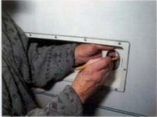
In my case, due to the positioning of the upper ventilator grill, I had to mark and cut the box so that it wouldn't obstruct the flue. Take care when handling the installation box as it is made from very thin aluminium and can be easily damaged.
