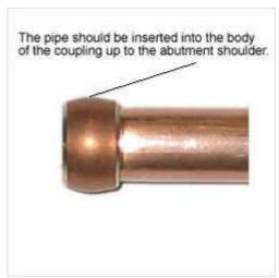
The coupling nut should then be tighten up by hand.
