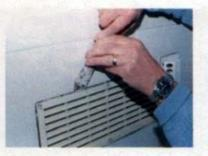
The heated blade will make cutting through the mastic seal easier.
