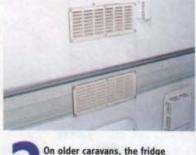
On older caravans, the fridge ventilator grilles are secured to the outer walls by screws.
