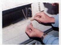
(Older grilles). Before refitting the grilles you must clean off all the old mastic. A piece of wood is ideal for removing most of the old mastic.
