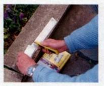
Once the grills have been refitted and secured by the screws, carefully trim off the excess mastic. Job done!
