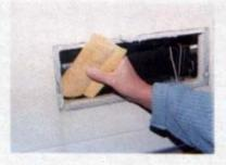
Use bits of rockwool to fill all the gaps that you can see between the rear of the fridge and the surrounding unit.
