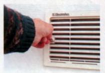
Turn the locking screw through 90 degrees to release the grille.
