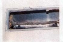
There should be some kind of heat baffle at the top of the fridge to deflect the heat out through the grille. If there isn't you may have to make one from thin aluminium. Sit it on rockwool along the top of the fridge.
