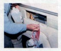
Remove the residual mastic with a rag dipped in Turps Substitute. Then thoroughly dry the whole area.
