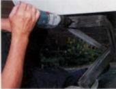
Although the holes are only 5mm diameter, you'll find it easier to drill them if you first make a pilot hole. Drilling underneath the caravan like this can be a bit awkward, so take your time and don't force the drill or you may break it.
