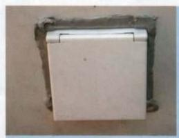
Having connected the cable from the consumer unit to the socket, I fixed the socket permanently in position, with the help of some mastic tape and screws that were supplied
