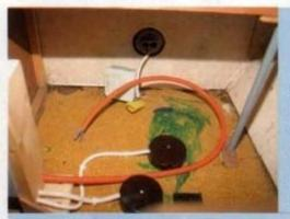
I had connected the consumer unit to two junction boxes, one cable being rated at 10 amp capacity and the other 6 amp. I intend to use the 10 amp for the mains sockets and 6 amp for lights and fridge
