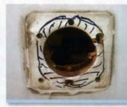
Having removed the old socket, I used the gasket supplied with the new socket to mark the enlarged hole which was needed. I then drilled some 6mm holes through the wall panel
