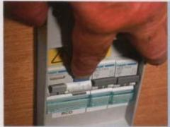
Once I had connected to the site mains, the next job was to test the trip on the RCD unit. As soon as I pressed the test button the unit tripped out, cutting power, so all was fine
