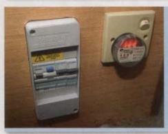
Having confirmed that the consumer unit was functioning properly, I checked that the 13 amp socket I had installed was wired properly, using my plug-in mains tester
