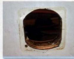
The old rule 'cut undersize and open the hole up' applied here. Having cut the hole undersize, I used my power file gradually to remove material until the socket fitted
