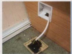
Having removed a continental-type socket here, I fitted a new mains socket. I ran cable round the van using some plastic ducting to protect it, seen on the left of the picture
