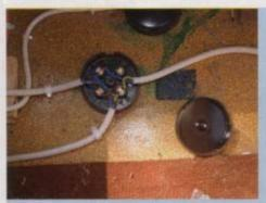
In the front nearside seat I connected the cable to the 10 amp junction box: brown (live) to brown; blue (neutral) to blue; and green/yellow (earth) to green/yellow
