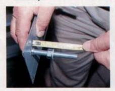
Having measured the thickness of the floor, fit the coachbolts through the holes in the top plate and run the nuts down them until the measurement from the underside of the plate to the washer is 2mm less than the floor thickness.
