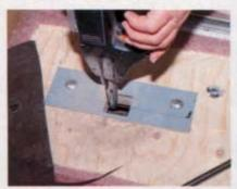
Carefully pass the coachbolts down through the floor and use a power file if necessary to open up the 50mm square hole to size. There is sufficient free play available to enable you to adjust the position of the top plate slightly.
