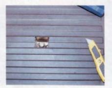
Replace the mat well, or other floor covering, and push a sharp knife down through the mat or floor covering as near to the centre of the square hole as possible – and then cut outwards to the edge to make an opening for the lock block.
