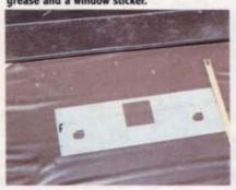
Place the top plate with the letter F facing forwards, in position so that the centre of the square hole is 75mm towards the inside of the caravan from the pilot hole. Use a tape measure to ensure that the plate is parallel to the doorway.
