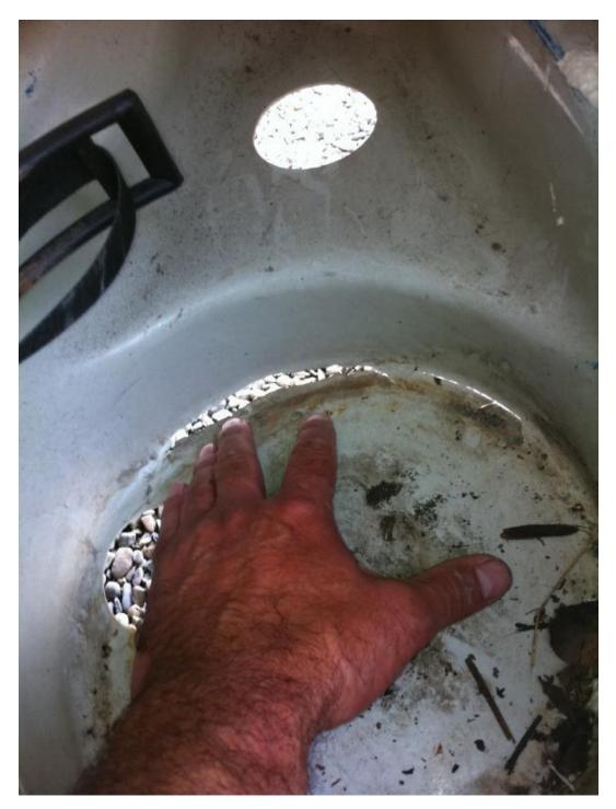
So my old skills at boat repairs have finally come in handy. I have made a GRP tray to sit inside the plastic liner to support the gas bottle.
