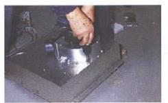
It's now time to think about fitting the heater, but first you need to punch out perforated knock-outs for the exhaust duct and air intake for the fan in the outer and inner installation box shells. Then assemble the shells using the five self-tapping screws provided. Finally, secure the fan unit to the outer shell with three screws.
