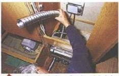
Feed the metal exhaust duct through the hole in the installation box and up to the exhaust cowl. This will give you an idea of its final length. Withdraw it and, having allowed for a small amount of excess, out it to length. Next, cut the outer insulation duct to the same length and fit it over the exhaust duct.
