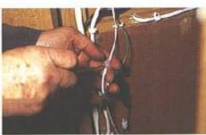
The mains control box should be screwed in position where it can be reached easily. The wiring instructions are clear and easy-to-follow. One cable plugs into the top socket on the Trumavent fan and connects to terminals 10 and 11 in the control box. Also on this plug are two short lengths of 12v cable. These will need extending to connect to an existing 12v supply. The lower socket on the Trumavent is for the cable which plugs into the fan control on the top of the front case.
