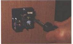
Drill a 10mm diameter hole through partition adjacent to the heater at a height the wall switch is to be fitted. Feed the 3-core cable though and then connect it to the three terminals on the switch. Secure the switch to the partition and refit the cover and control knob. The cable is pushed through the entry at the left-hand side of the control box.
