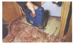
Drill 10mm diameter holes in the corners of the cut-out and use a bradawl to pre-start the five holes for the heater's fixing screws. Then use a ligsaw to cut the opening.
