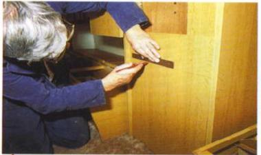
Carefully mark the cut-cut for the heater, 465mm high x 480mm wide.
