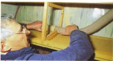
Run the ducting to the outlets, cut it to length, and push it into the outlet.
