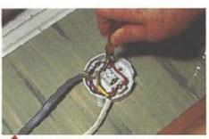
The maximum output of the heater on electricity is almost 9 amps. If possible, it should be connected to its own 10-amp circuit in the consumer unit. If this isn't possible, cut into a suitable circuit at a convenient point and fit a junction box. Connect a length of 3-core cable with a minimum 10-amp rating to the junction box.
