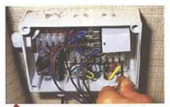
From the junction box, run the cable to the control box. The cable enters via the right-hand entry and connects to terminals L1, N, earth. Use cable clips to secure the cable at intervals.
