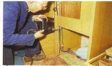
Cut the opening slightly undersize and use a file or powerfile, to open it to the correct size.
