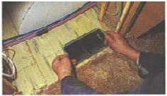
Insert the half frames into the opening and use small screws to secure them in position.
