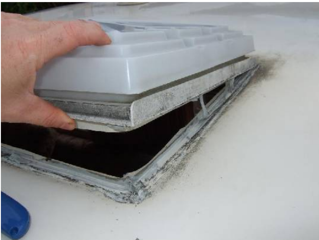
Once done, you can gently prise the old roof vent up
