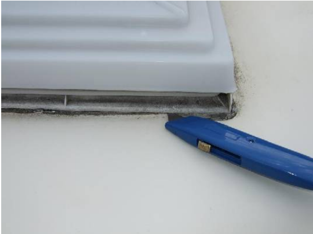
Outside, you need to carefully cut around the old mastic
