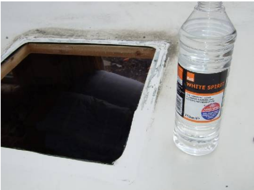
White spirit will dissolve any remaining mastic. I used plenty of kitchen roll to wipe off the excess.
