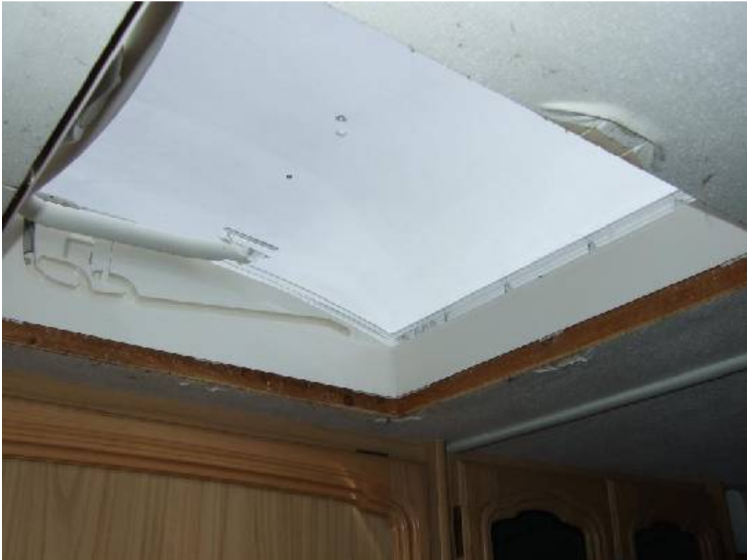
Inside, the vent is ready to receive the inner surround
