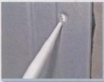
Before screwing the panel back into place I placed a blob of silicone sealant in the hole so the screw would seal when fitted
