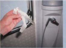
I used masking tape to protect the shower room walls while applying flexible sealant, after re-fixing the unit. You must remember to peel the masking tape off before it sets
