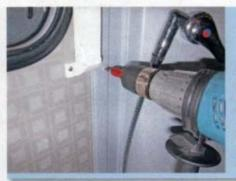
I removed the screws holding the shower head unit in place but found that the Dometic cassette blind would have to be removed as well. This will involve removing the fixing screws...
