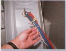
While the unit was off I tidied up the wiring by lightly strapping it to the water pipes with cable ties. This ensured that nothing would get trapped when the unit was refitted
