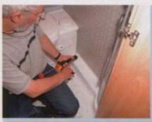
I then extended application of silicone away from the shower head unit to cover any areas into which water might run
