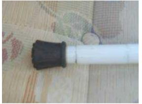
A rubber foot is fitted to the base of the leg to stop it cutting into the carpet or flooring of the van. These can be purchased from most DIY stores.
