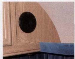
The speakers are fixed in place by four screws each (supplied). Once they're in position you simply push-fit the protective grilles into the surrounds. Take care when doing this to avoid denting or otherwise damaging the grilles. The cables can now be secured in position, using either Superglue or cable clips.
