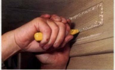
... I could use a Stanley knife to cut the actual opening for the unit. I then used a power file to finish the edges of the aperture neatly. Obviously you can use an ordinary file if you don't possess the powered version.
