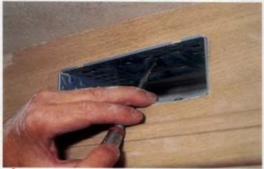
Having pushed the mounting frame into position in the opening, the next thing to do was to bend the locking tabs outwards with a screwdriver to fix the frame securely in position. You need to be quite firm when doing this but you should take care not to push too hard or clumsily and distort the whole thing.
