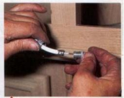
The next job was to cut the co-ax cable to the right length and fit a plug to the end. Don't worry if you've never had to fit a plug to a coaxial cable before – the instructions on the packaging are extremely clear and easy to follow. If, however, you are fitting a new aerial, it makes sense to take care of installing that before cutting the cable.
