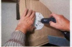
Using the template supplied with the loudspeaker packaging, mark the positions where the speakers are to be fitted. But before drilling the pilot holes for the cutter, check inside your lockers to make certain that there are no obstructions, etc that might cause problems.
