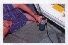
2 Drill the 6mm hole for the cable up through the floor only after making sure you've chosen a suitable spot.
