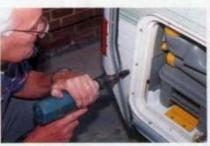
3 Cut the socket hole through the side using an 11/16" hole cutter after careful marking and positioning.
