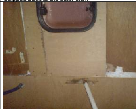
New plywood attached to fill the 'gap'
