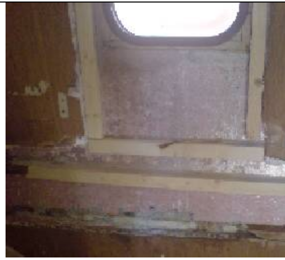
New battens stuck into place.
