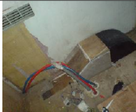
The new marine ply cover and cables now back in order.
