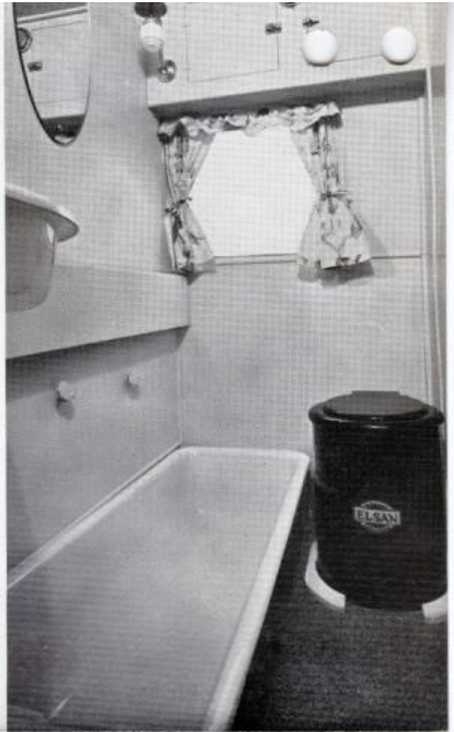
Bathroom : With wash basin, → perspex bath and chemical toilet.
